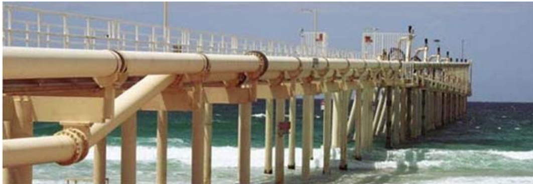
Figure 10. Trestle of Tweed River Sand By-pass System 13
