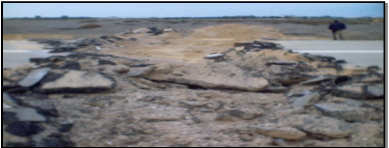
Deep bulldozing of the runway
